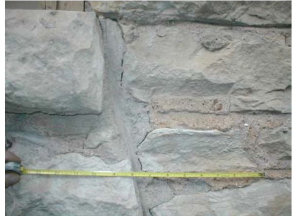
Exterior Flexure Cracks (under windows near the left tree)
