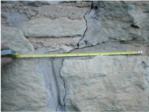
Exterior Flexure Cracks (under windows near the left tree)
