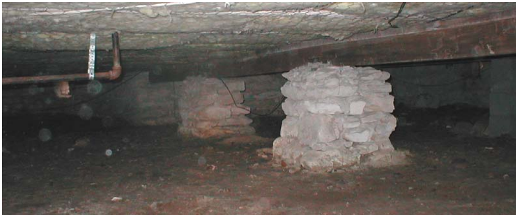
Original (masonry) Post Supports at Main Beam
