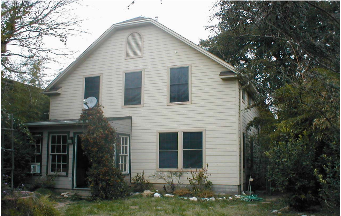
Rear Elevation (addition and converted porch)
