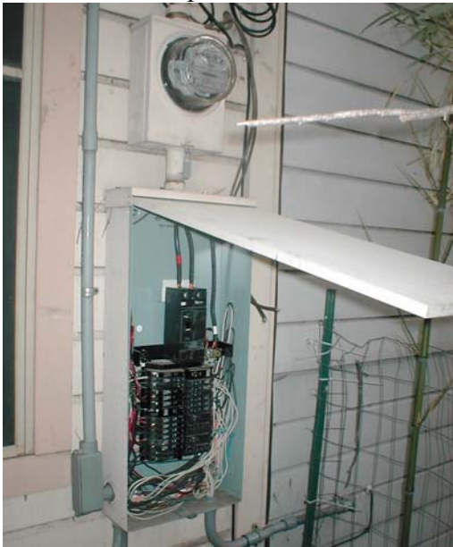
Exterior Service Entrance (right wall)
