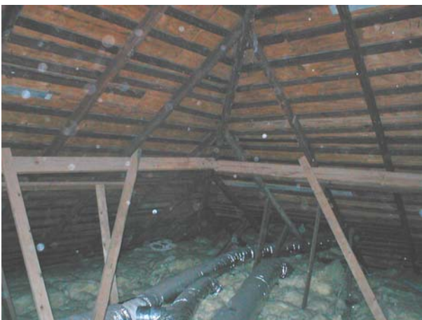
View of Main House Attic (very over-spanned)
