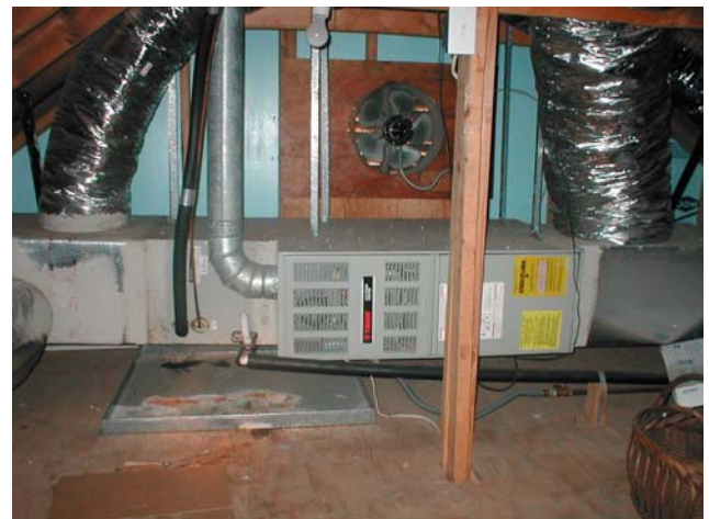
Upper Fan-Coil-Furnace
