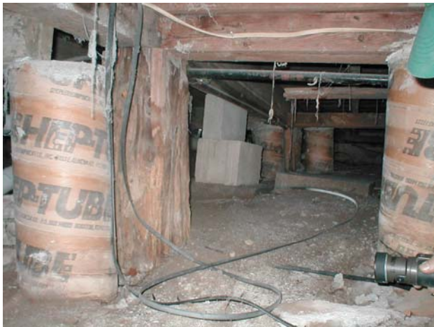
There are a lot of improvised supports in this crawlspace.
