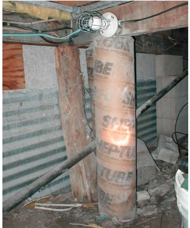
View of Beam Connection Support (rear, left side)
