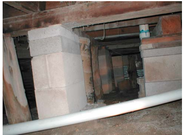
There are a lot of improvised supports in this crawlspace.
