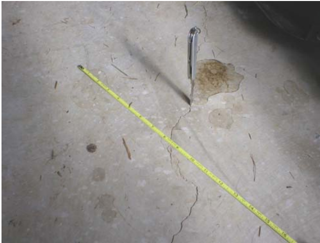
Shrinkage Cracks (at garage floor surface)
