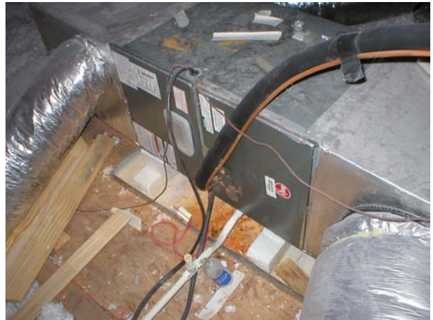
Furnace-Fan-Coil (attic)
