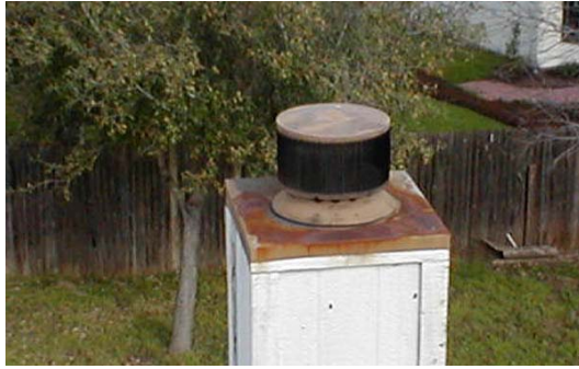
View of Chimney Crown (from roof)
